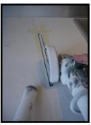
7.Cut along the two lines up to the holes, use a vacuumed to prevent dust
