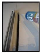
11.Apply a waterproof flexible sealant to edge of cut out
