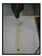
6.Drill a 10mm dia. Hole ate each end
