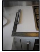
3. Position knife slot and ensure it is square and aligned
