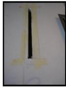
8. Remove the cut out and vacuumed up the dust
